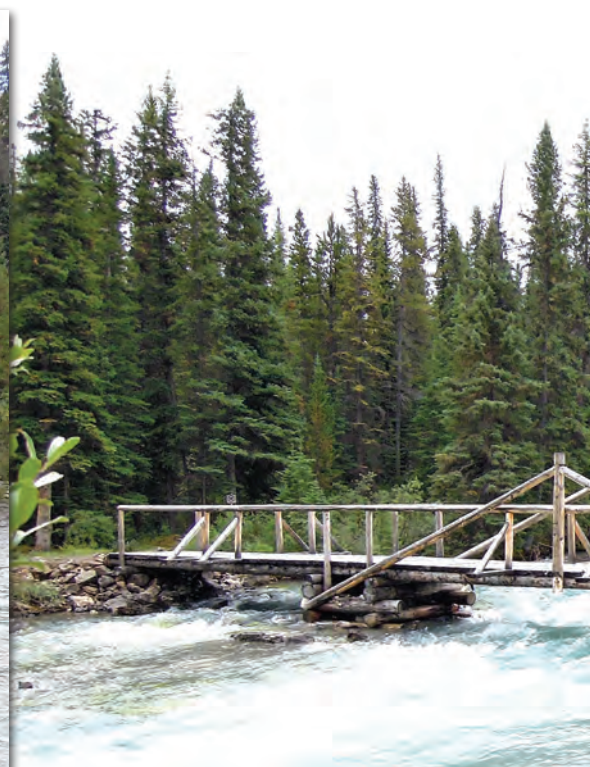
The Brazeau River dropped 0.6 metres or two feet from its flood levels in July, allowing a safe crossing.
